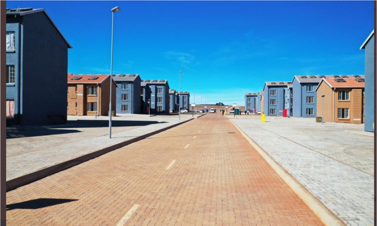
Elijah Barayi Mega Human Settlement Development in Merafong – Completed and allocated units
