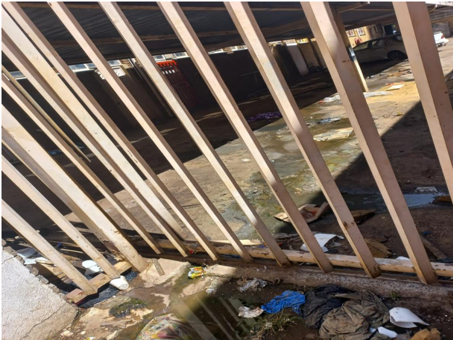
Unhygienic condition in a privately owned premise
